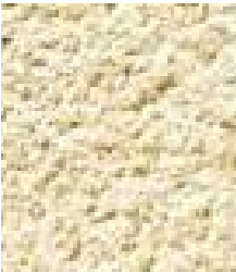
Finish :- Painted Texture Sand /Cement Render
